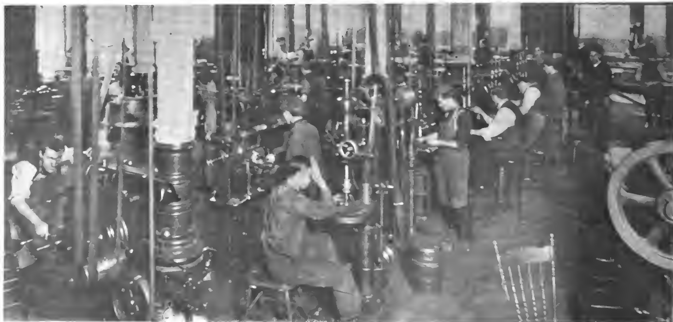
One of the Work Rooms in the New York Plant Where the Herz Specialties are Made.
